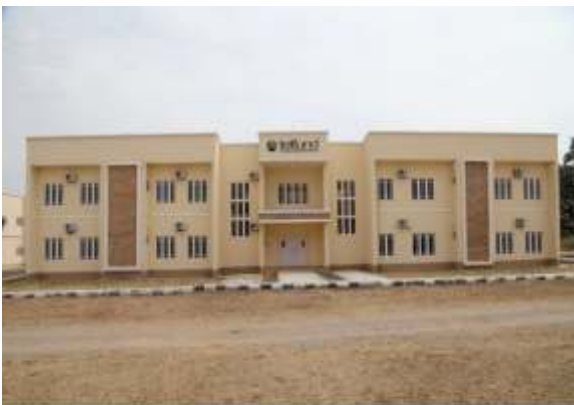
The Departmental Building Block E, at the Abubakar Tafawa Balewa University, Bauchi State.
