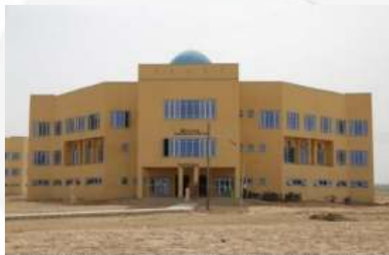
The School of Secondary Education Business, at the Federal College of Education (Technical), Bichi Kano State.
