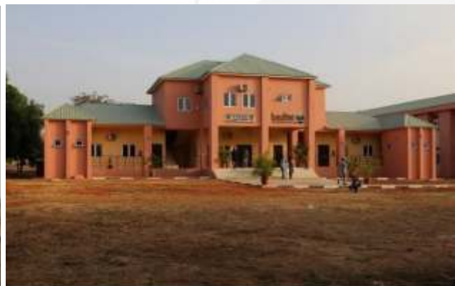
Department of Cyber Security building at the Nigeria Defence Academy (NDA).
