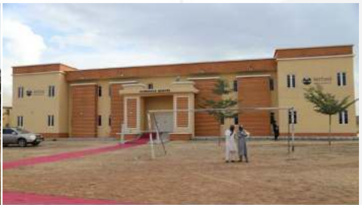
The Students' Hostel Block, at Abubakar Tafawa Ali Polytechnic, Bauchi State.
